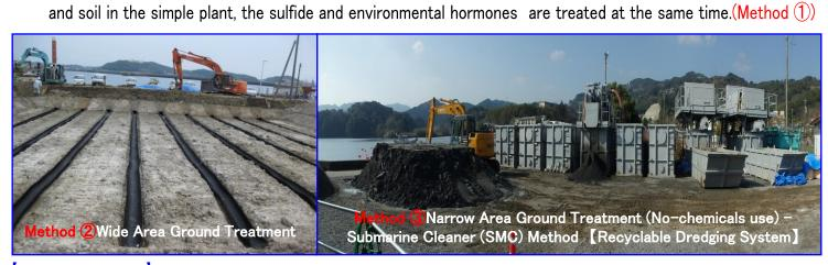
[Recyclable Dredging System] The sea water after removed of sand and silt in the ground facility will be reused for the injection water of Submarine Cleaner.
